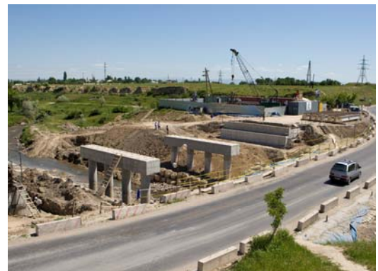
The bridge construction process
