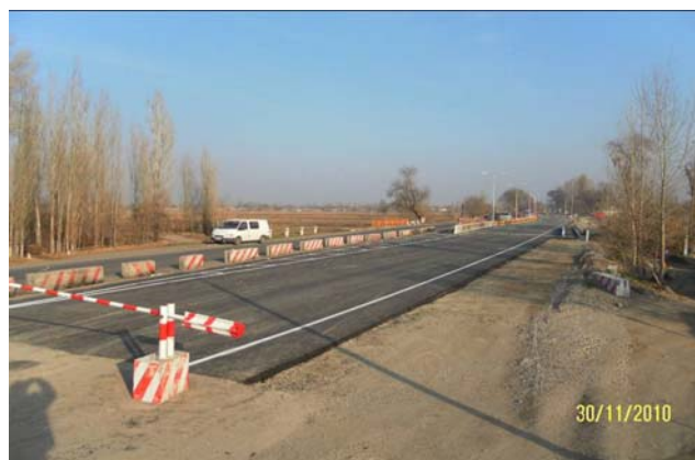
Bridge over the Ken-Bulun river after reconstruction
