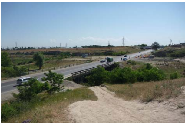
Bridge over the Alamedin river before reconstruction
