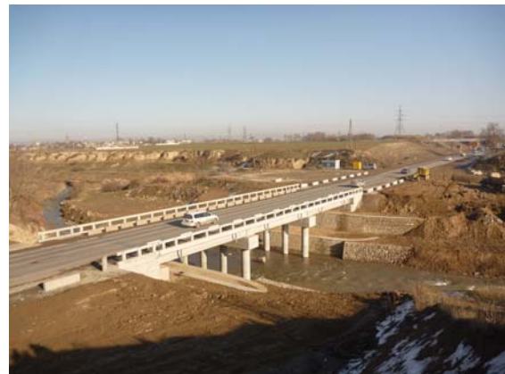
Bridge over the Alamedin river after reconstruction
