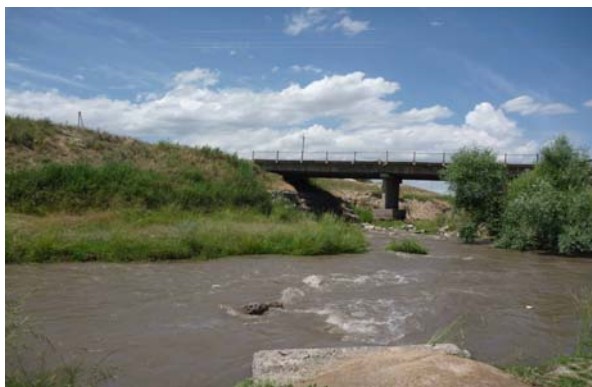
Bridge over the Ala-Archa river before reconstruction
