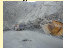
Dangerous part of the road
